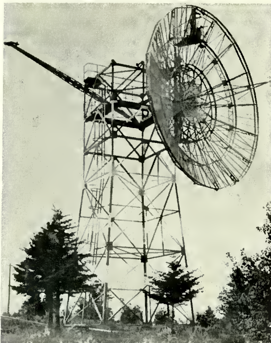
Fig. 4—Transmitting antenna installation at Covey Hill.
